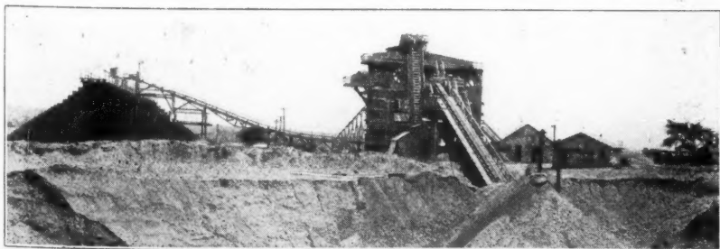
View Looking at the Plant From One End of the Deposit
